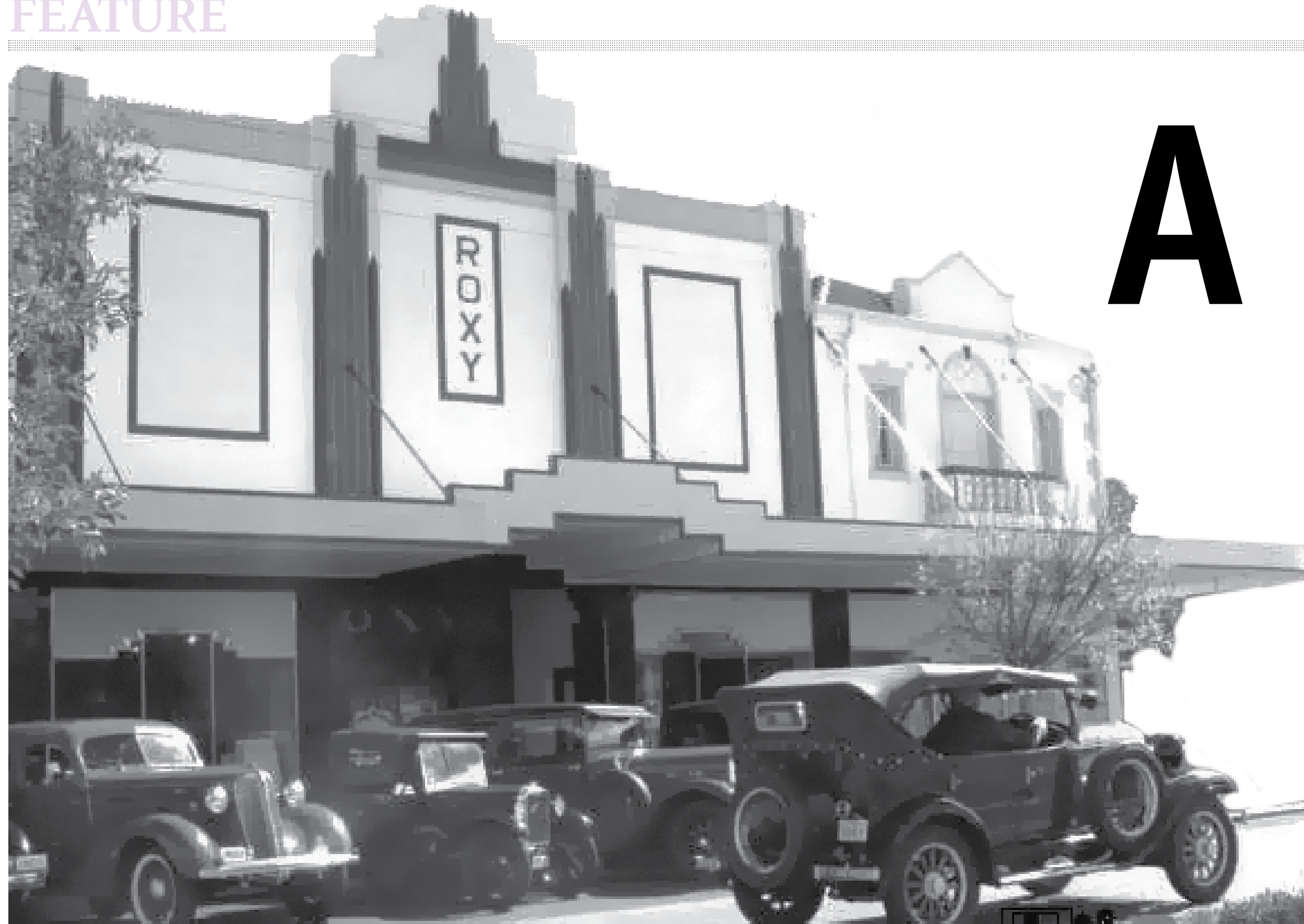
The original facade of the Roxy.
